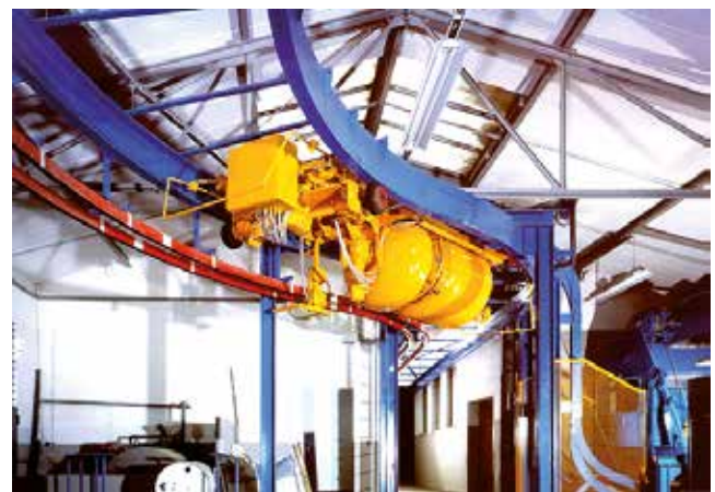
Feed and control of a concrete skipper
