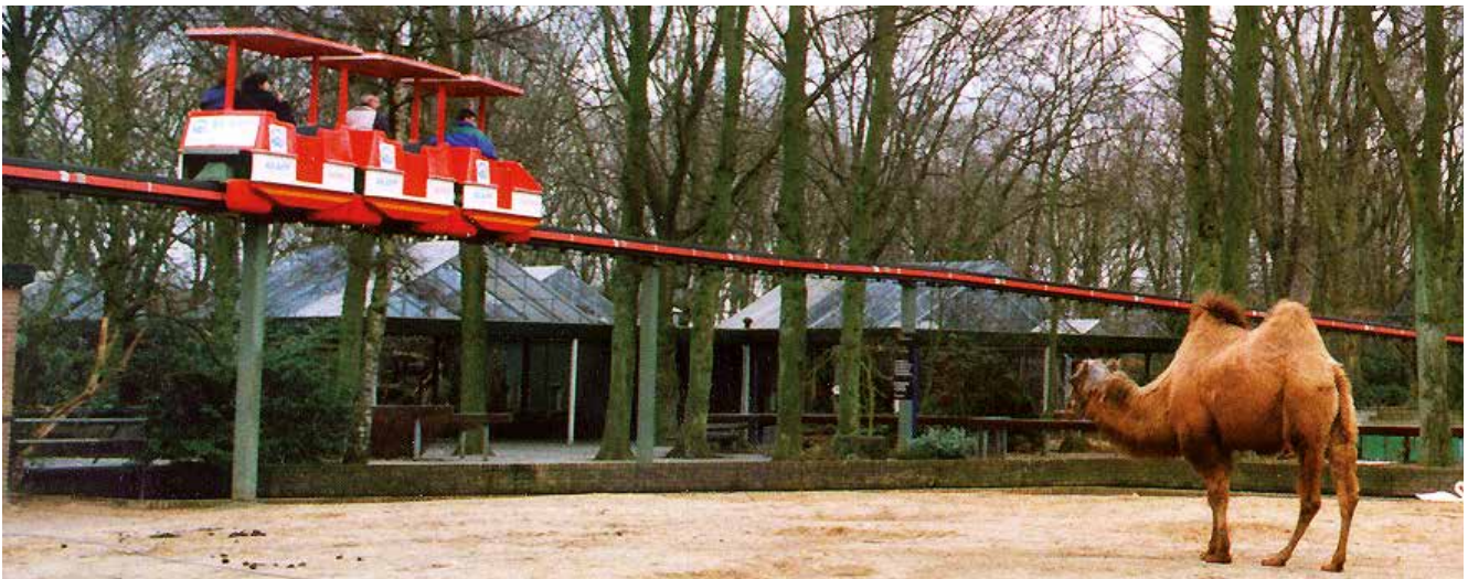
A 500 m long enclosed track for a passenger train in the zoo
