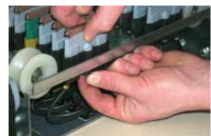
Replacing the carbon brushes.
