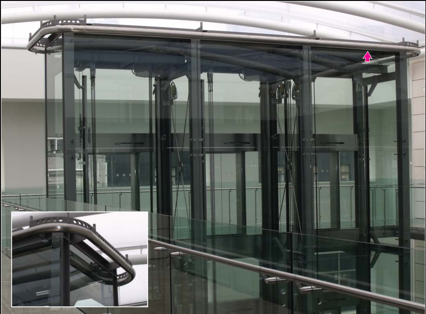
Tracks can be installed as either soffit or face mount and in both cases the main supporting structure can be fixed back and concealed within the building structure.
