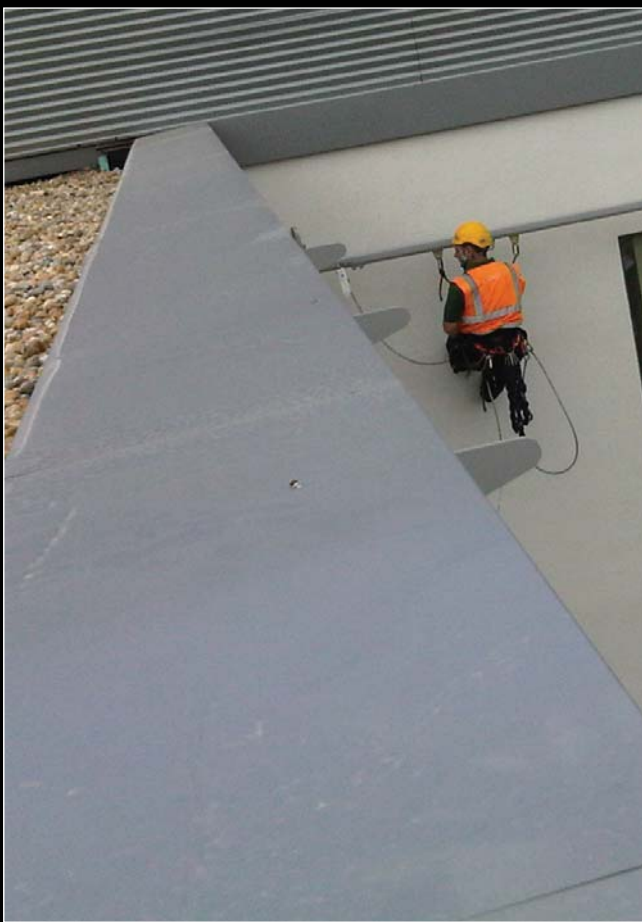
Tracks can be installed as either soffit or face mount and in both cases the main supporting structure can be fixed back and concealed within the building structure.
