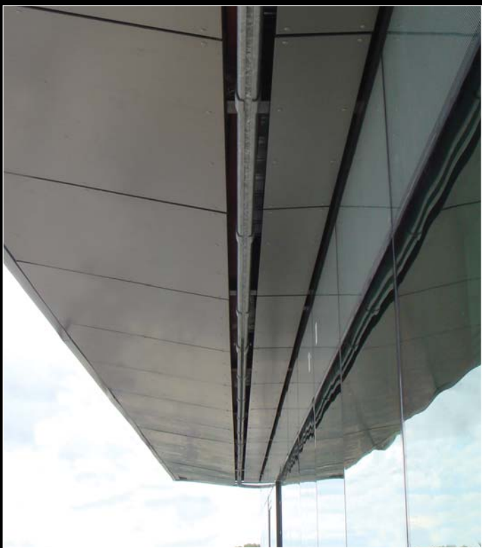
Tracks can be installed as either soffit or face mount and in both cases the main supporting structure can be fixed back and concealed within the building structure.
